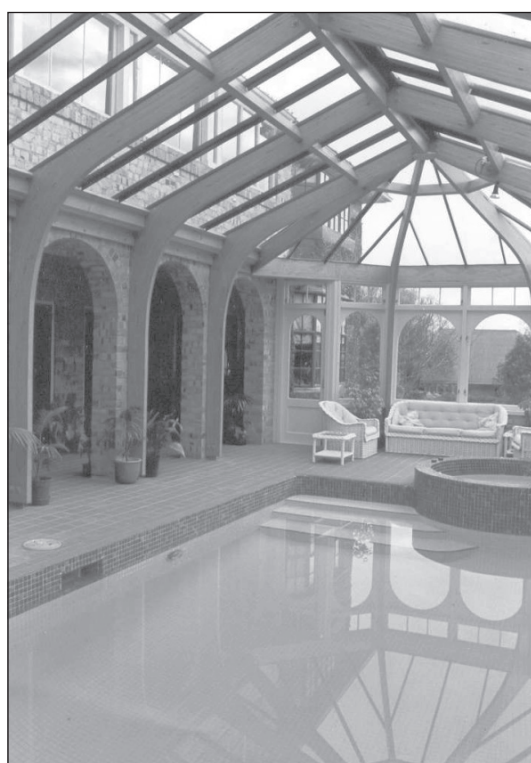
Curved Glulam portals highlight the design flexibility and natural beauty timber can bring in an indoor – outdoor situation.
